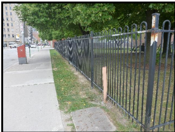
Image 33: Area of Surficial Potential (August 28, 2018; Facing Southeast)
